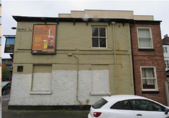
(Side Elevation from Brindle Street)
