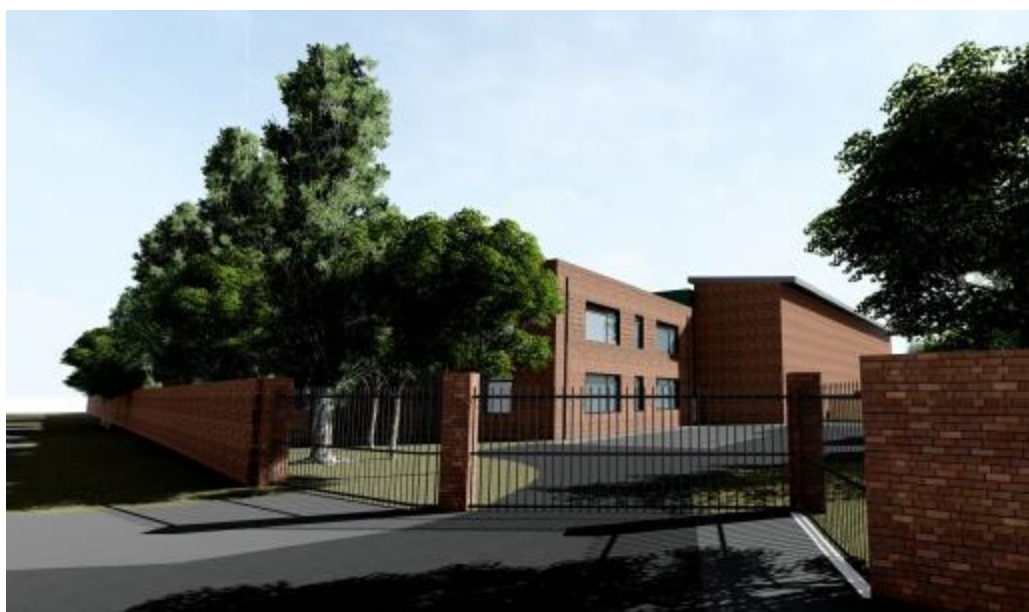
CGI of the proposed building as viewed from Dagenham Road
